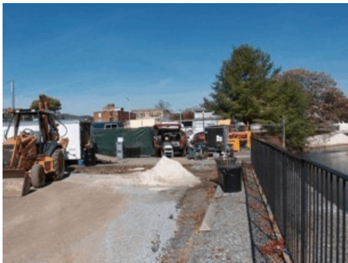
Figure 2. Open-Path FTIR Spectrometer at the Bristol Site Cleanup
